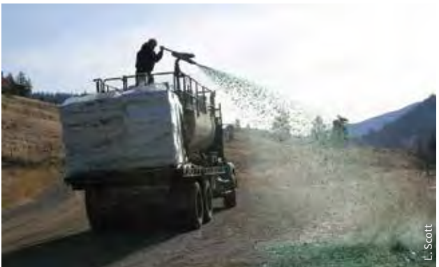
Hydroseeder at work.
